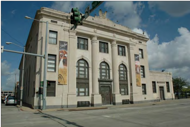
This is a Classical Revival Style commercial building with a temple front form.
