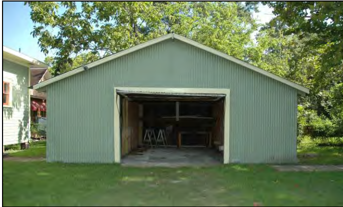
Example of a detached garage.
