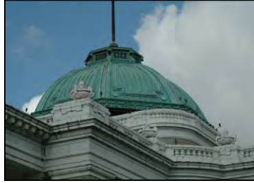
On this Classical Revival government building, the molded cornice, roof balustrades, and dome are important character-defining features.
