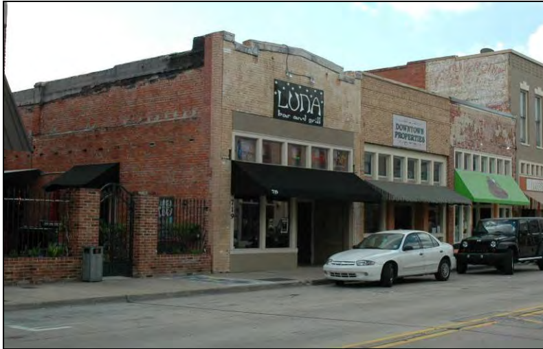
A grouping of Prairie Style one-part commercial block buildings. Note the storefronts, transom windows, and parapets.
