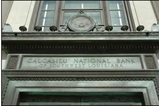
When signage is integral to the original design and materials of a building, it should be maintained regardless of changes in tenancy or use.
