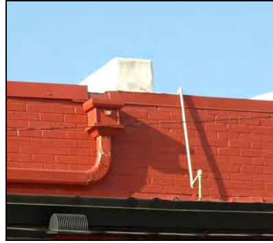
This building's mechanical equipment is inconspicuously mounted on the roof to minimize visibility from the street.
