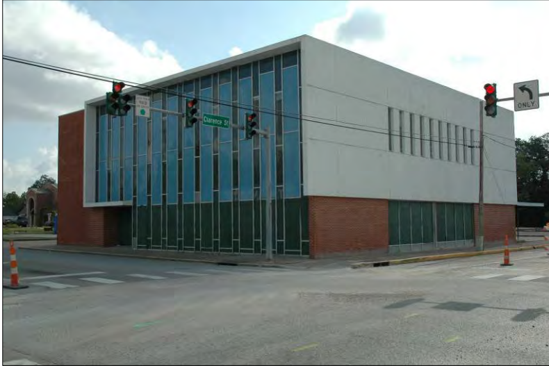
A Modern commercial block building.
