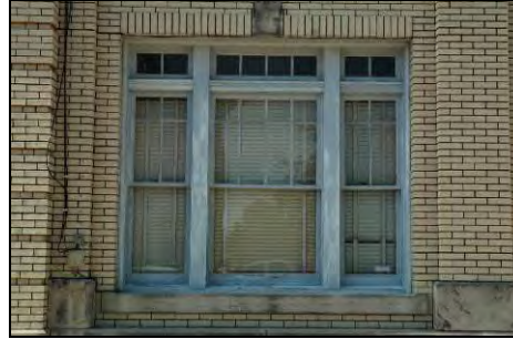
The geometric grid of muntins and number of lites in this building's double-hung windows are character-defining features.
