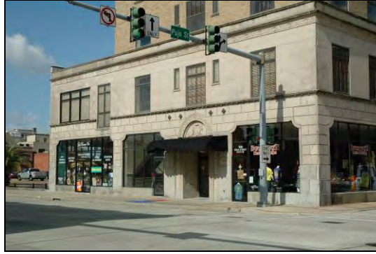
The storefront in this three-part vertical block is emphasized by larger windows, a recessed entry, different wall materials, and ornamentation.
