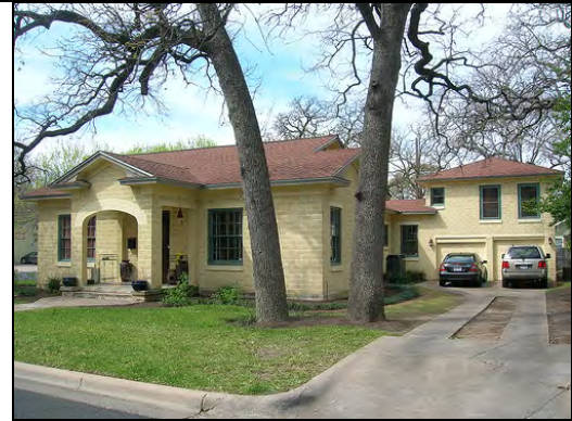
The addition is set back behind the original rear façade and does not destroy or detract from the character-defining features of the original building. The materials and windows used are in keeping with the original building.
