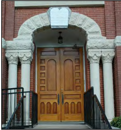
The rusticated door surround with column supports and paneled wood doors are character-defining features of this Romanesque Revival building.
