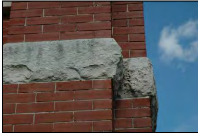
The character of an exterior wall is defined by its texture, color, and pattern. Note use of brick and stone string course.
