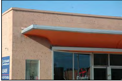
The paint color and curved edges of this cantilevered canopy are character-defining features of the building's Art Deco Style.
