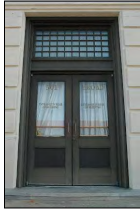
Note the proportions of the doorway and of the glazing to the wood.
