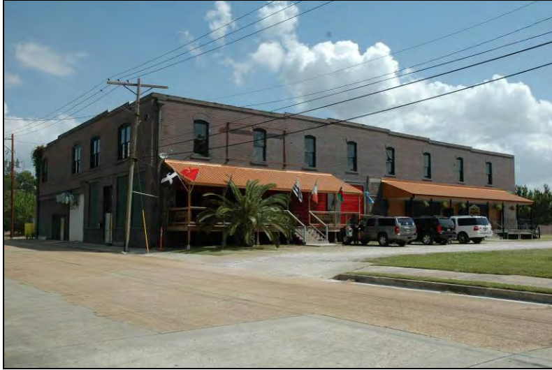
Example of a warehouse. Note loading bays.
