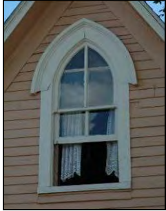
Note simple molding and divided lites at this Gothic arch window.
