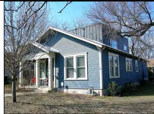
The addition is set forward almost flush with the front façade of the original building. The flat roof is not compatible with the character of the original building. Modern or Contemporary design may be appropriate for an addition, provided that it is not visible from the street.
