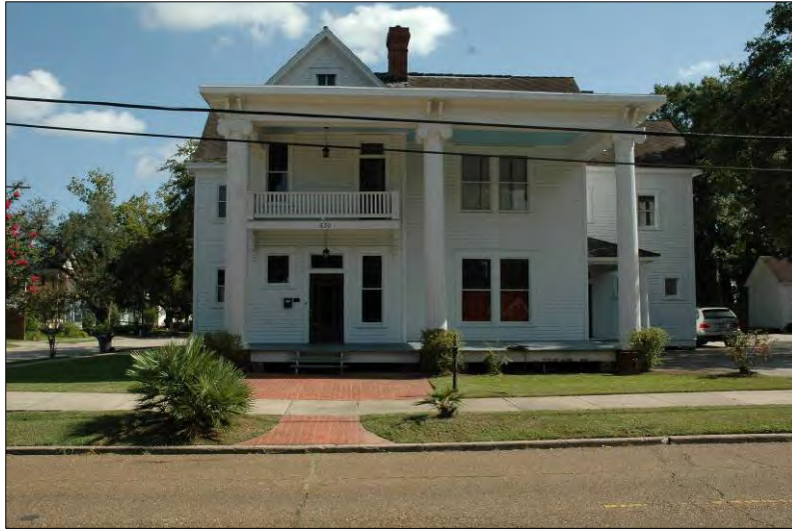
Example of a foursquare Classical Revival house with a rear addition. Note the porch with monumental columns.
