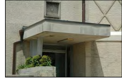
This concrete cantilevered canopy is consistent with the use of materials in this building.
