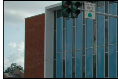
Use of multiple materials is a character-defining feature of some buildings. Note the glass and ceramic spandrel curtain wall.
