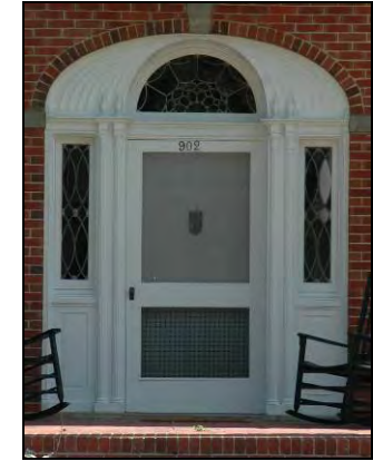
Note the segmental arched surround framing the door with sidelights and fanlight.
