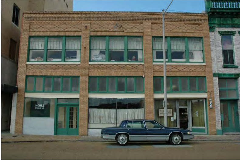
Example of a Prairie Style two-part commercial block. Note geometric detailing and storefronts.
