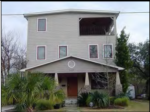
The addition is set forward flush with the front façade. The three-story scale overwhelms the original building. The roof form and fenestration pattern do not reflect the character of the original building.
