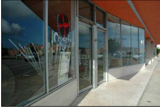
Note the proportion of glass to metal in this storefront's doors and windows, as well as the terrazzo flooring at the entry.
