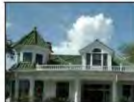
The green tile roof, cornice, balustrade, and varied roof dormers are character-defining elements of the Queen Anne Style.
