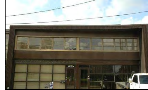
The casement windows at the storefront and ribbon windows in the transom complement the façade of this enframed wall Modern building.
