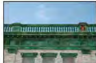
The terracotta roof parapet with balustrade and cornice is an important feature of this Italianate commercial building.
