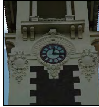
As an important mechanical feature, this historic clock on this building has been maintained.
