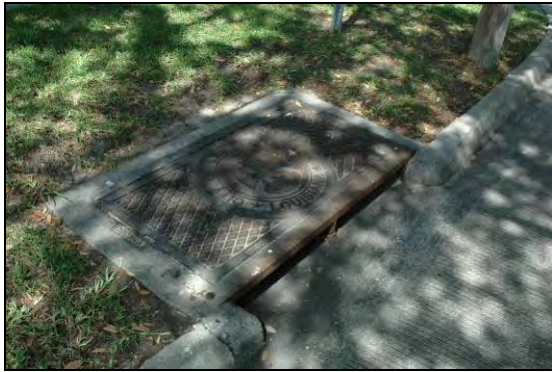
Infrastructural elements, such as culverts, are character-defining features of the streetscape of historic districts.
