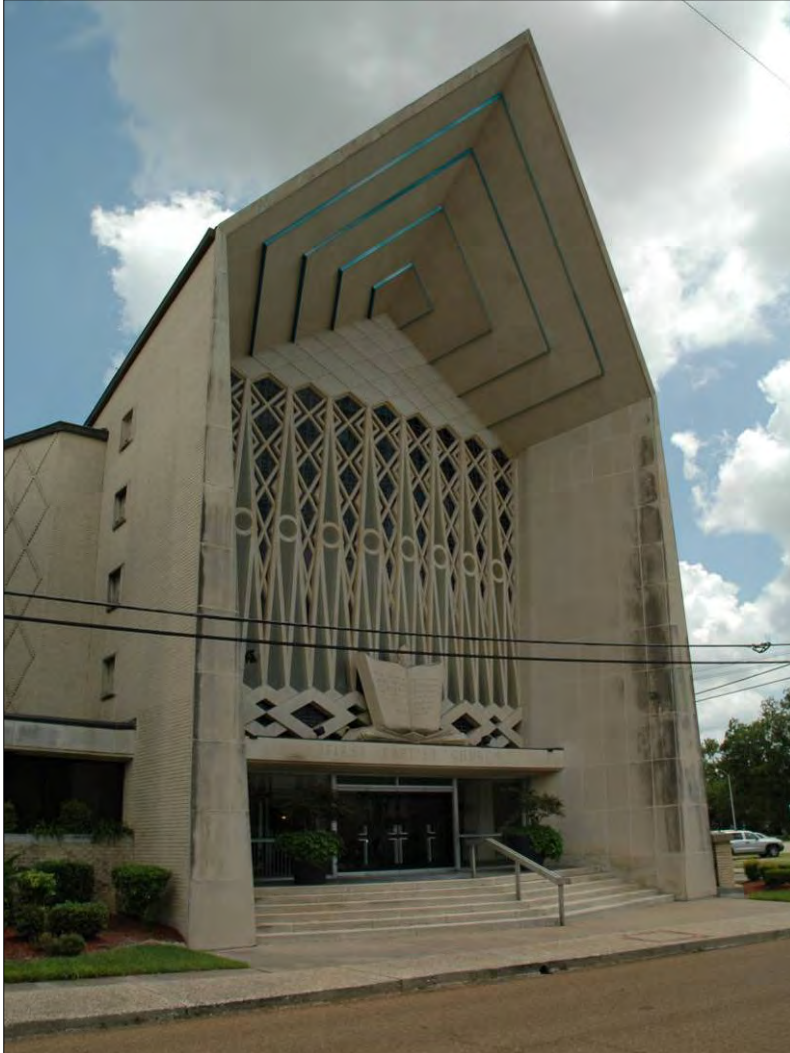
A Contemporary Style church. Note the cantilevered canopy over the entry and the angled end walls.
