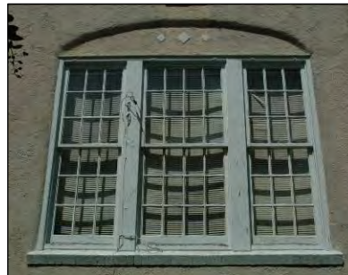
The geometric grid of muntins in these windows is characteristic of the Spanish Revival Style.
