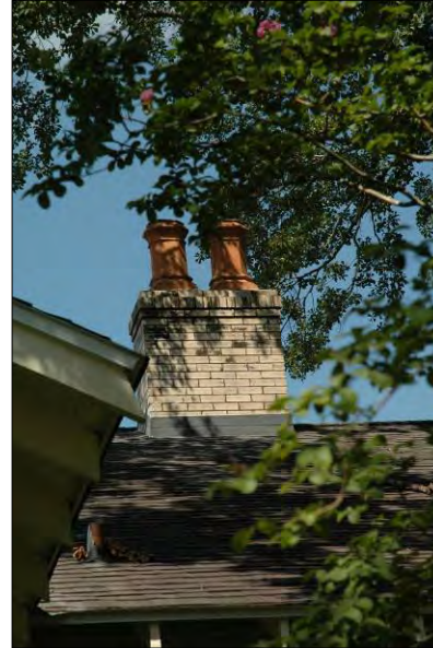
The terracotta flues are character-defining features of this chimney.
