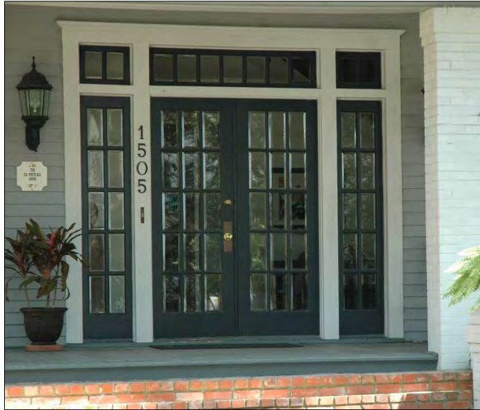
The sidelights, transom windows, and double doors are character-defining features of this residence.
