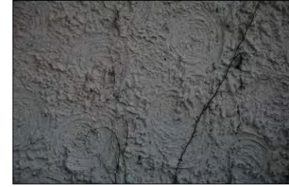
The exterior stucco with its swirl patterns is a character-defining feature of this residence.
