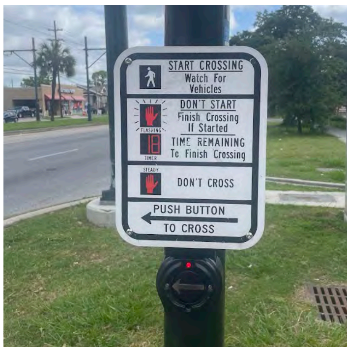
Pedestrian push button with audible feedback. Lafitte Greenway, New Orleans. Credit: ATG/DCCM 2024
