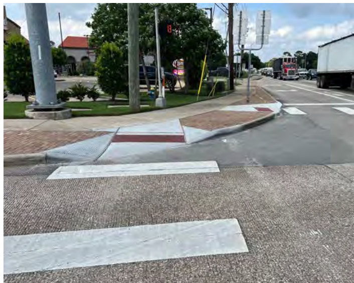
Curb ramp at intersection in Pearland, Texas. Credit: ATG/DCCM 2024
