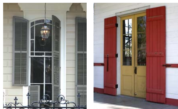
Doors and full-height porch windows increase ventilation
