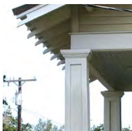
Half-Height Tapered, Paneled Box Column on Pier
