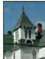
Note pyramidal roof, brackets, and eyebrow dormers at this tower on a home with Queen Anne elements.
